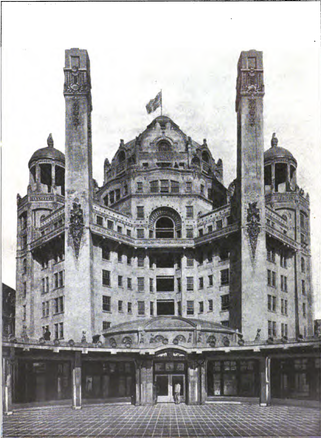
Abb. 24. Marlborough-Blenheim-Hotel in Atlantic-City, N.-J., V. St. v. Amerika. Haupteingang. Arch. Price u. Mc. Lanahan.
